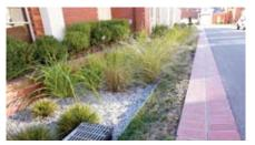
A rain garden is a specially designed garden bed that takes rainwater directly from a roof or any outdoor surface that produces run-off. It has a sand base and can be planted with a range of plant species.
