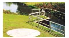
Gross pollutant traps are intended to retain litter, debris, and in some cases sedimentation, from stormwater systems primarily through screening and rapid sedimentation, without considerably retarding flows.
