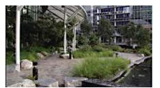
Constructed wetland systems use sedimentation, fine filtration, and nutrient-uptake processes to remove pollutants from stormwater. Constructed wetland systems generally consist of an inlet zone (sediment basin to remove coarse sediments), a macrophyte zone (shallow heavily vegetated area), and a high-flow bypass channel.
