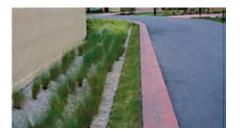
Vegetated swales are used to convey stormwater in lieu of pipes. The system uses overland flows and mild slopes to slowly convey water downstream. The interaction with vegetation facilitates pollutant settlement and retention in the vegetation. Vegetation acts to spread and slow velocities, which in turn aids sediment retention.
